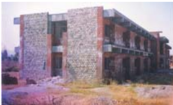
Dormitory Under Construction
